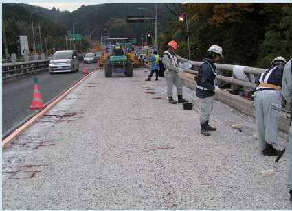
(床版切削状況)
